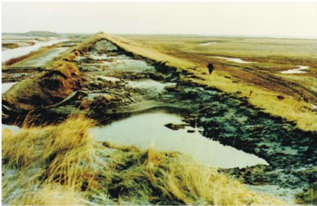
Fig. 4: Breach in an old dike
