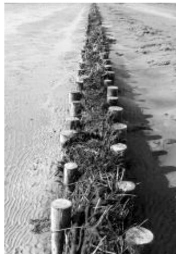
Fig. 1: Characteristic Natural Foreland and Cross-section of a Brushwood Fence in Northern Germany
