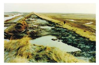
Fig. 4: Breach in an old dike
